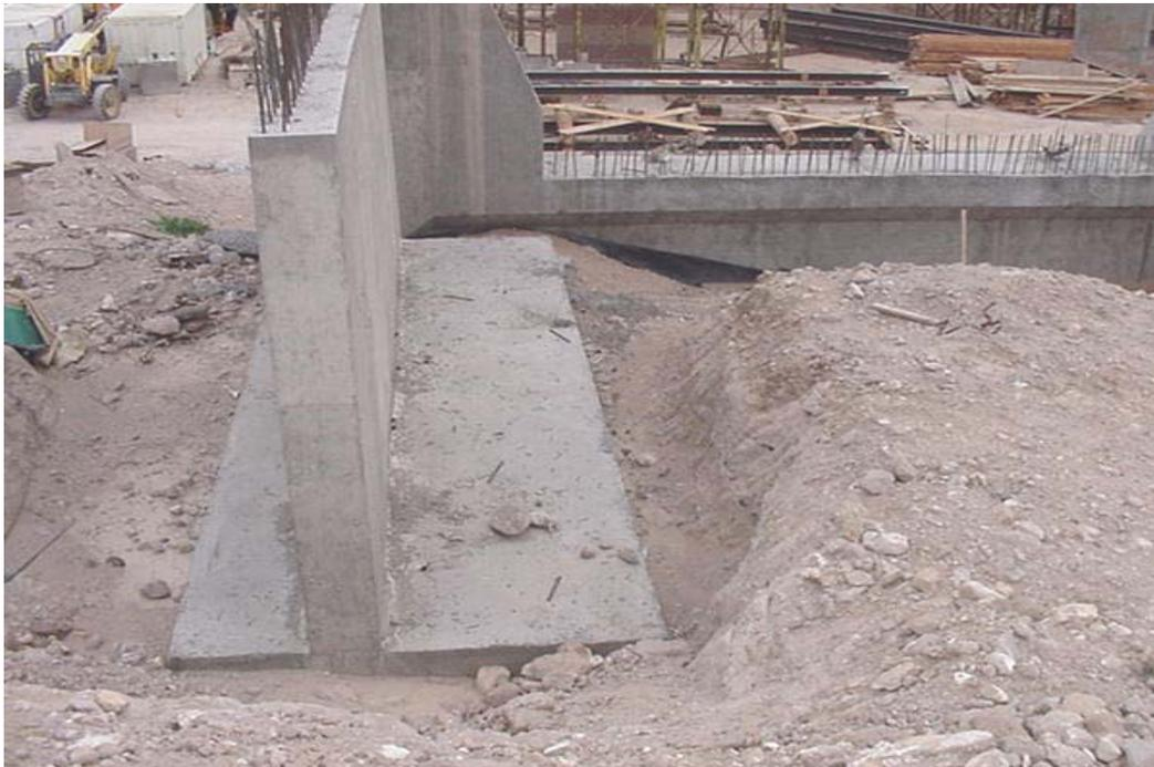
**Figure 8-5. Abutment/wingwall footing, I-10, Arizona.**
