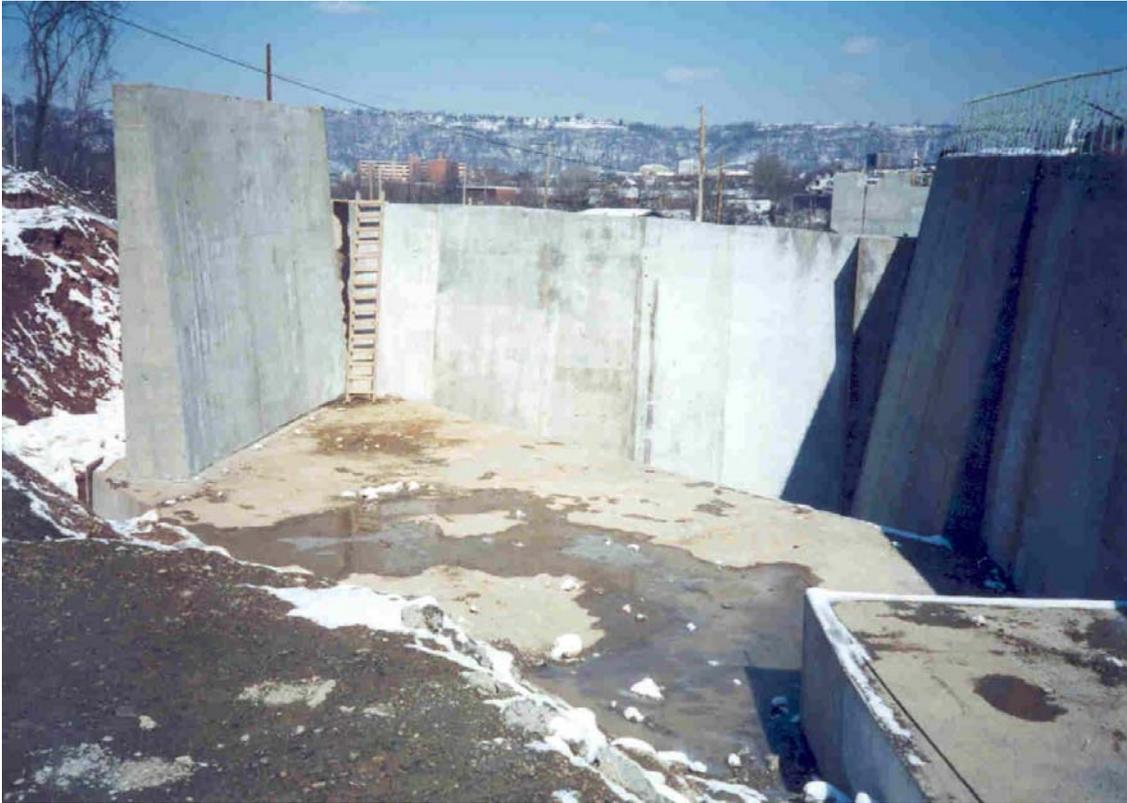
**Figure 10-18. CIP abutment with integral wingwalls**
